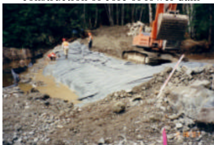
Figure 3, Lining core of dam with PVC liner
