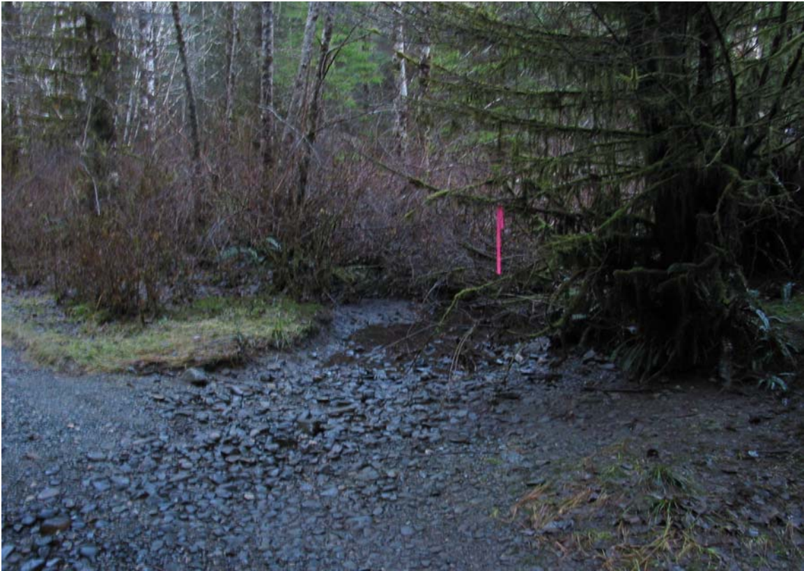
Photo 3: The lower swales where they cross the main access road.
