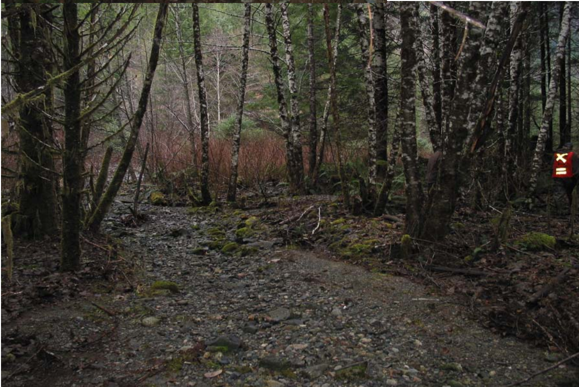
Photo 14: Gravel transport down the laterally unstable channels on the unnamed tributary alluvial fan. This source of sediment will have to be incorporated into the channel design.
